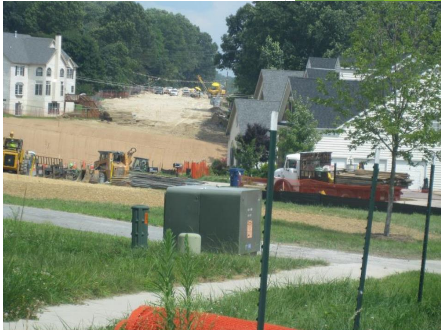
Chester County Residential Pipeline Worksite 2008
