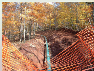
Pipeline in trench
