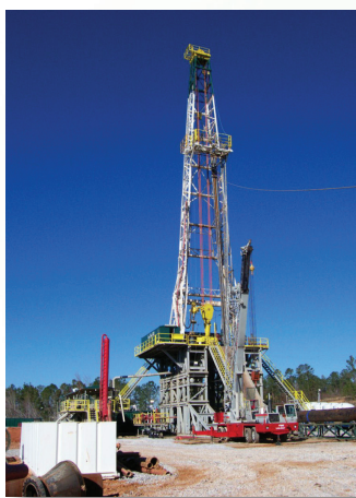
Well drilling rig
